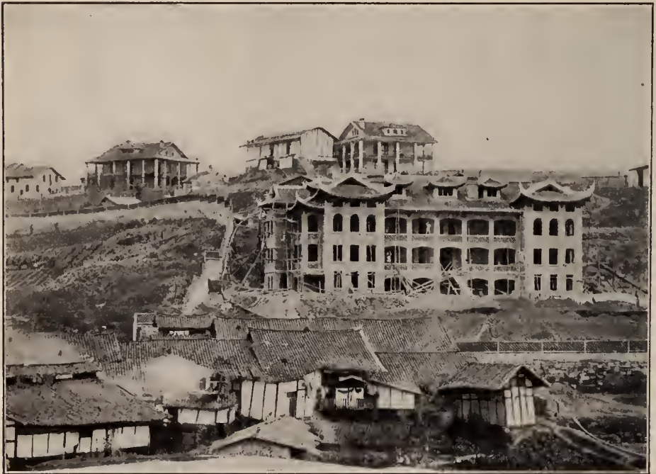
A MODERN MISSION HOSPITAL, IN CHINA IN PROCESS OF CONSTRUCTION
